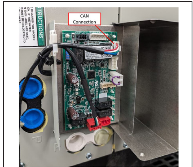
Figure 20: Comm/Link harness connection to MCB
