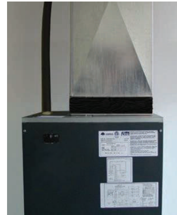
Figure 5. Prevent Transmission of Vibration
